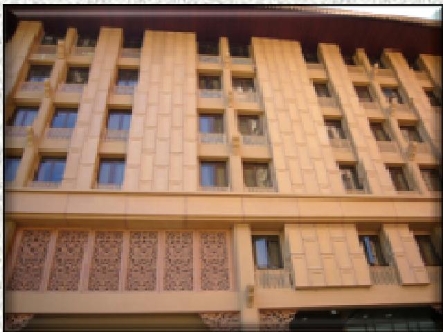
GFRC cladding offers numerous benefits to the architect, contractor and owner over other types of cladding or curtain wall.
